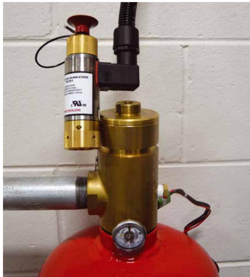
mechanical discharge of the extinguishing agent that will combat the fire.
